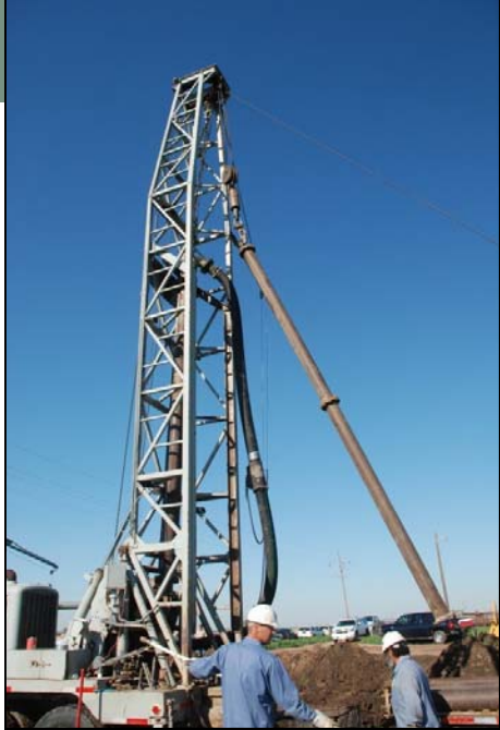
Drilling an Irrigation Well using a Reverse Circulation Rig
