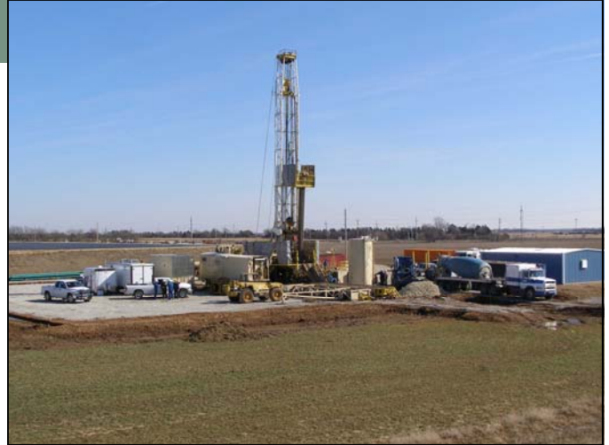
Drilling of New Hydrocarbon Storage Well
